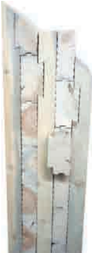
Figure 1: ICLT sectional profile illustrating a 5-layer system utilizing tongue and groove and dovetail joinery for structural capacity. This ICLT uses standing dead beetle kill pine from the intermountain west forestland.
