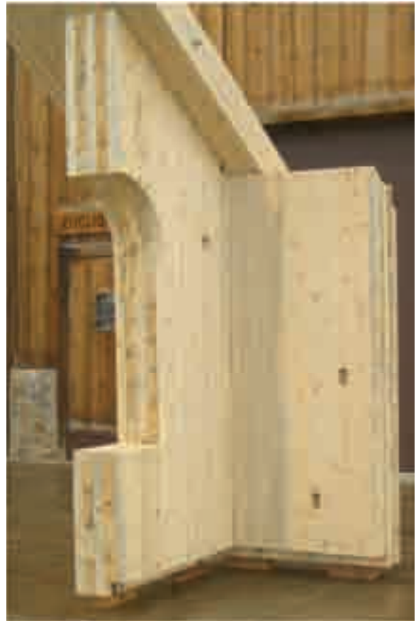
Figure 3: ICLT mockup of corner and roof connections.
