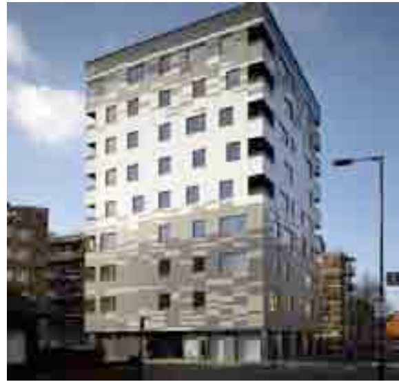
Figure 2: Nine story Stathaus Building in London designed by architect Andrew Waugh completed in 2009 is the world's tallest and largest CLT structure.
